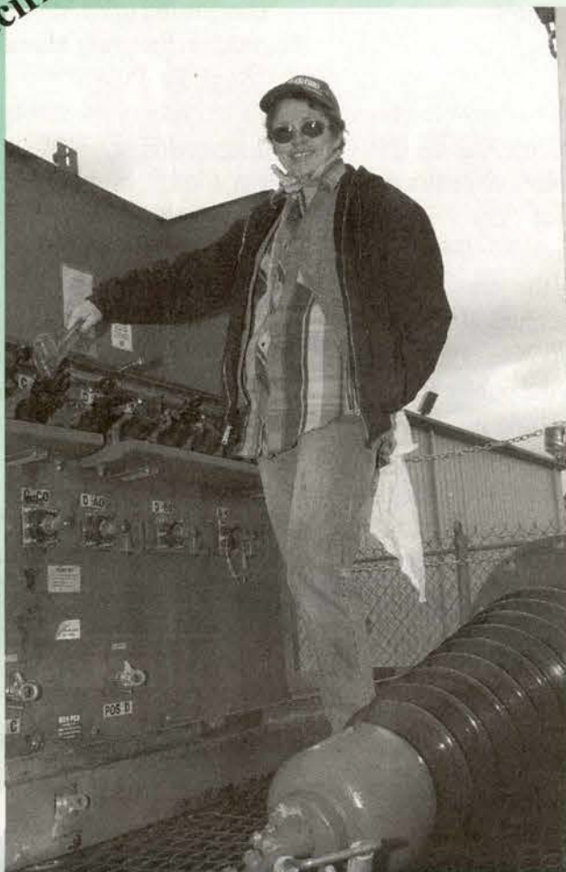
Sierra Pacific Power UMS Linda Stanley drains oil out of a switch in Reno, Nev.
