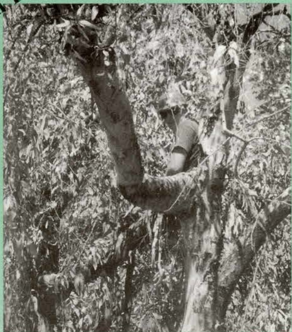
Second Step Line Clearance Apprentice Dennis Keithly, Asplundh Tree Expert Co., gets tough with some eucalyptus trees growing into a 12 KV line in Lucerne, Ca. (Lake County) last September.
