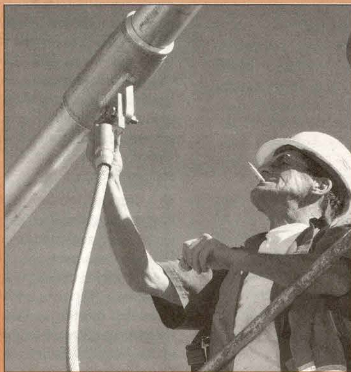
Lineman Ron Barrette bolts the jumpers.
