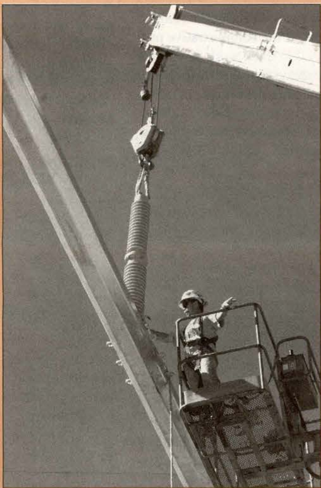
Lineman Philip Hamblock installs glass for the jumpers.
