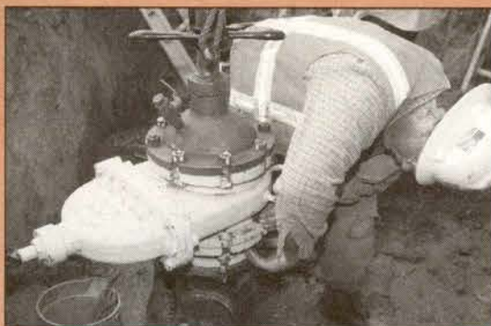
Jim Conroy installs the bolts to hold nine-inch gate valve on pressure control fitting.
