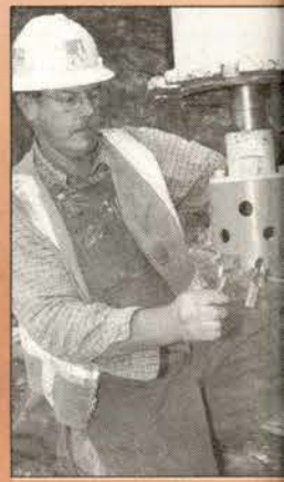
Jim Conroy lubricates six-inch shell cutter before taping out pressure control fitting.
