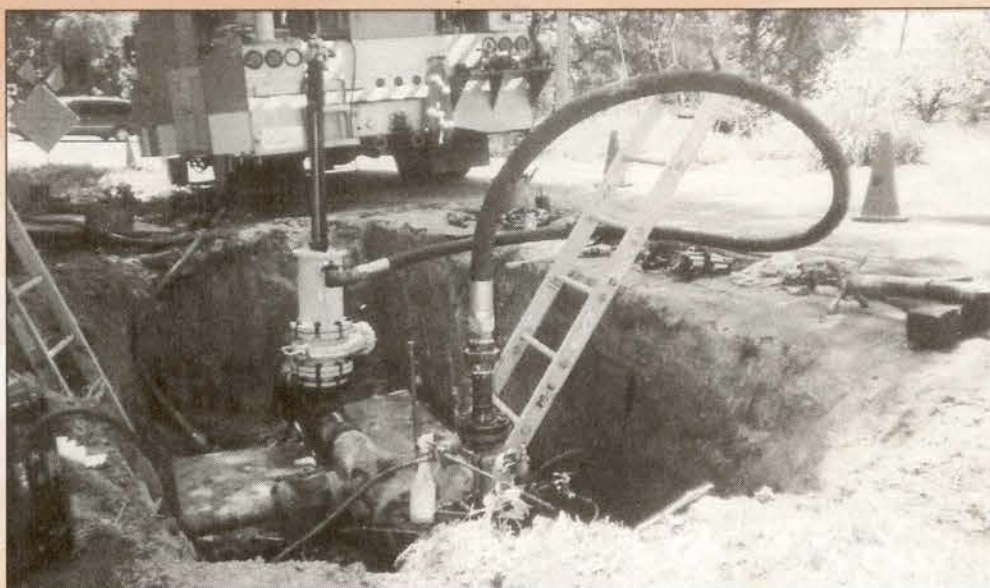
Six-inch plugging unit with high pressure by-pass and regulator.
