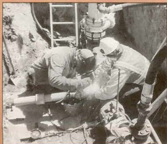
Jim Conroy and Richard Peter weld in new three-inch valve.
