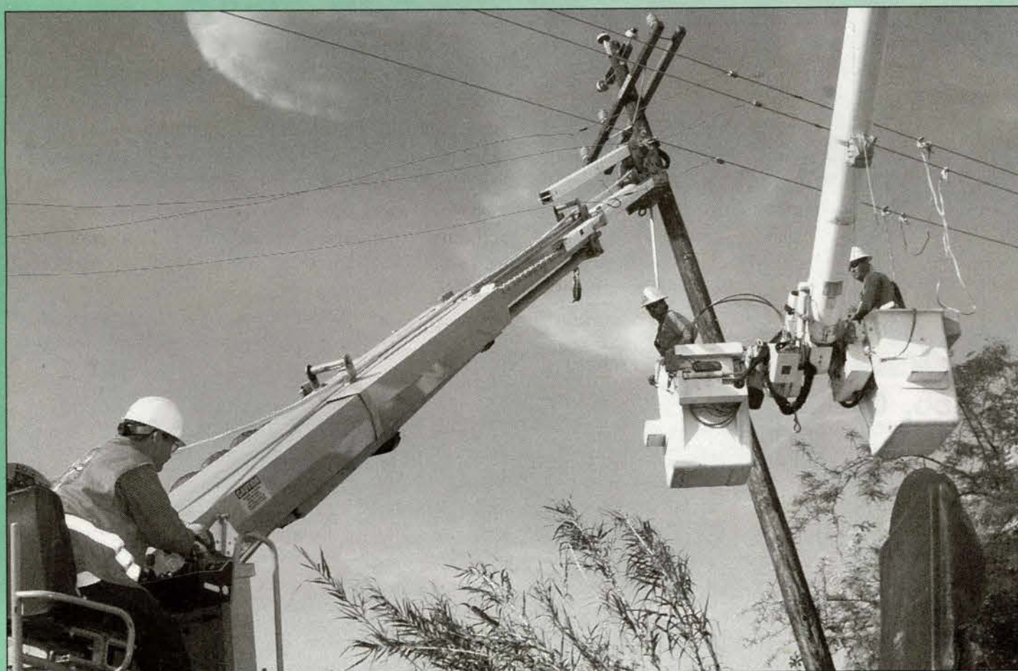
Foreman Lucky Carter (left), Lineman Dave Kelly (in bucket, on left) and Apprentice Lineman Jeff Gomes.
