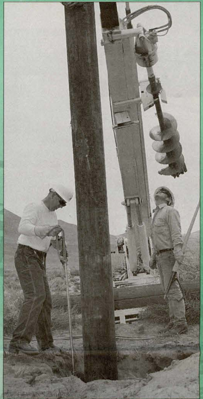
Apprentice Linemen Brad Shell (left) packs dirt around the pole.
