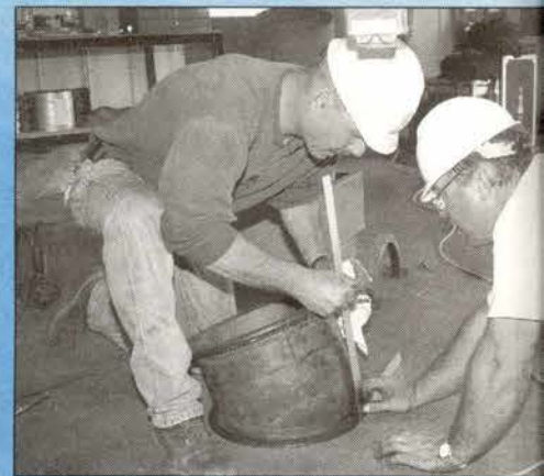
Bob Ballew (left) and Frank Rutledge find center so the combustion piping can be re-
