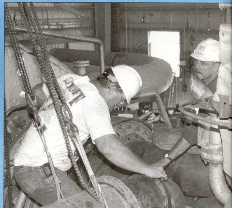
Frank Rutledge (left) and Bob Ballew install combustion piping on t
