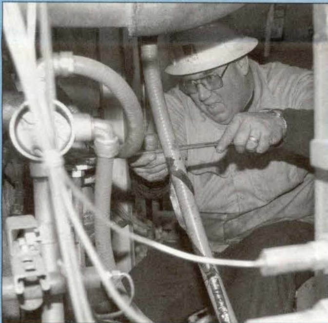
Jeff Wilson changes out rubber boots on a frame 3 lube oil drain on a GE turbine.
