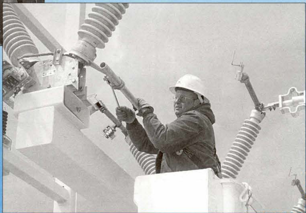
Tom Cornell puts final adjustments on switch.
