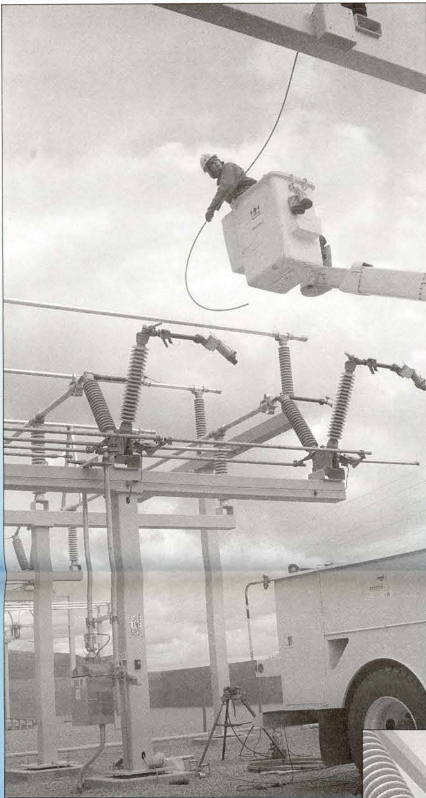
Randy Brunelli installs jumpers.
