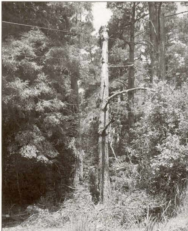
An enormous "spar"—a tree with the limbs removed—is left standing at a private residence in Fort Bragg. The removal form said the entire tree was to be removed, but Family Tree never finished the job. "Eventually that thing is going to fall down," says union tree trimmer Carl Lamers.
