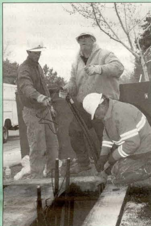
Sean Cherry, Mike Armstrong, and Steve Curl guide the old cable as it is pulled out of the ground.
