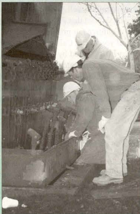
Checking the damage are Mike Hillyer, Sean Cherry and Mike Armstrong.
