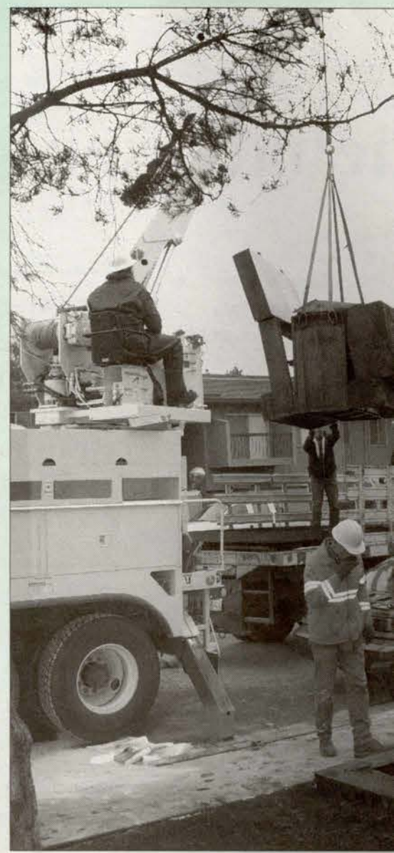
The ruined transformer is loaded onto a truck to be inspected.
