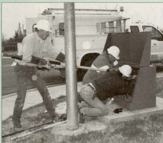
Foreman Steve Curl, left, and Troublemakers Ron Frugoli and Javier Garijo work a switch across the street in an effort to restore power.
