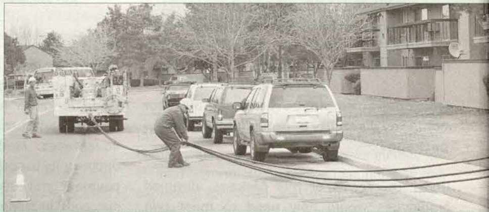
Using a truck to pull out the old cable.
