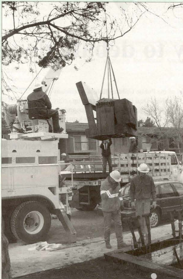
The ruined transformer is loaded onto a truck to be hauled away and inspected.
