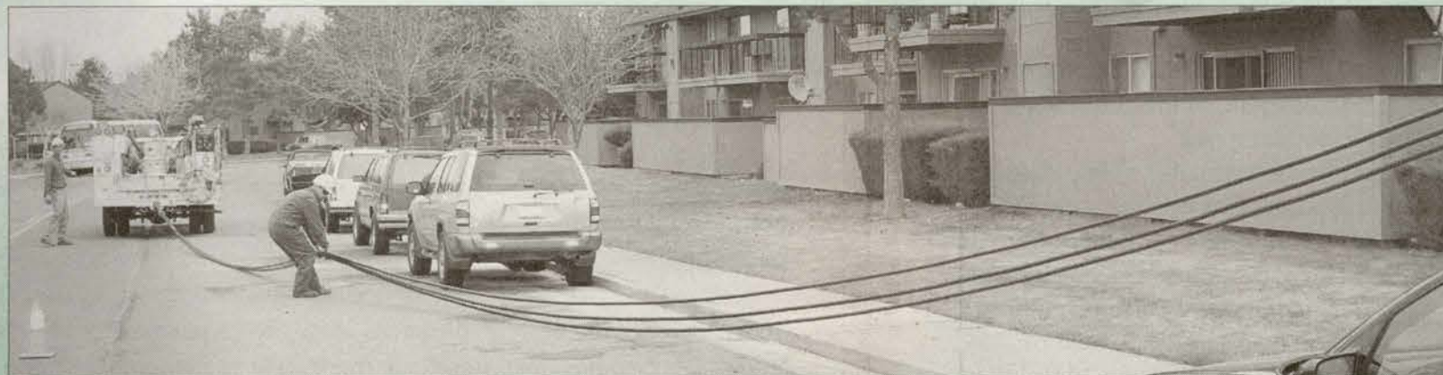
Using a truck to pull out the old cable.
