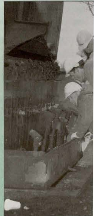
Checking the damage at the scene. Sean Cherry and Mike Armstrong
