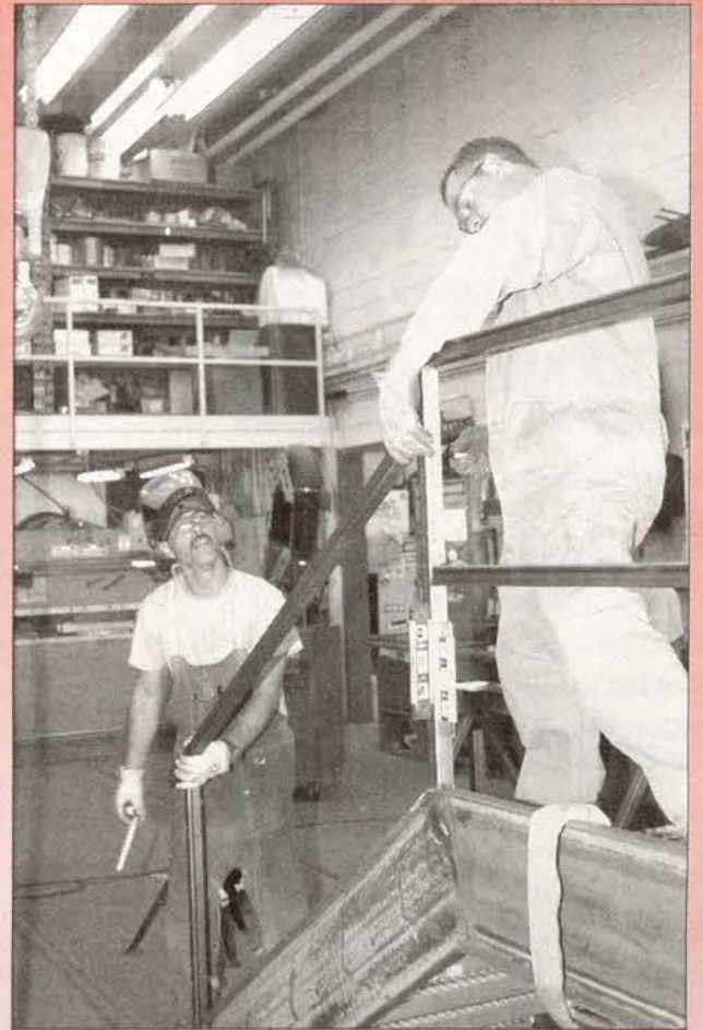
John Jackson (left) and Dan Haskill build a stairway for going over gas pipes at Tracy Power Plant.
