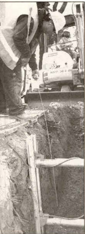
Utility Worker Rolando [unclear] measures if [unclear] are deep enough.
