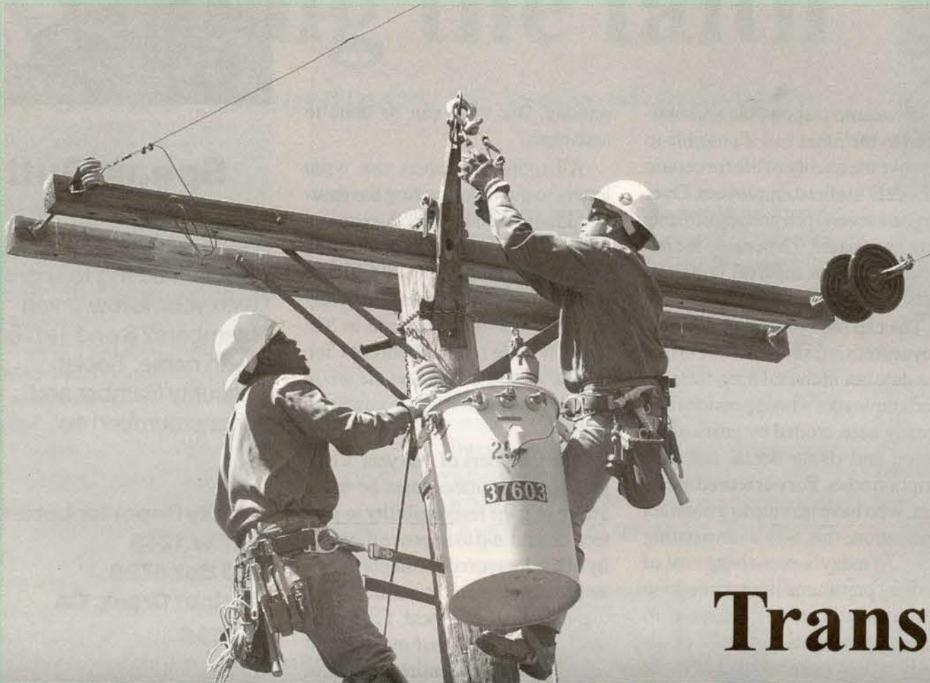
Linemen Reggie Slayton (left) and Steve Bancroft remove the old transformer.
