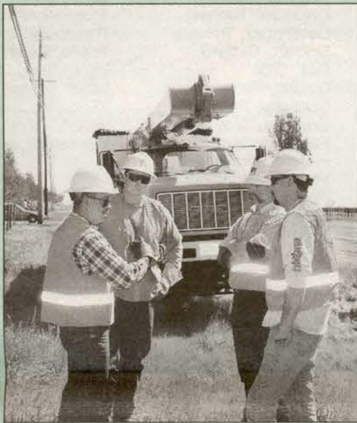
At the tailboard in preparation for pole replacement are, from left: Electric Crew Foreman Ray Rendon, and Linemen Jeremy Lehne, Vick Mahafley and Steve Hernandez.
