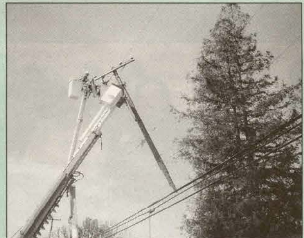
Pole grabbers used to lift damaged pole out of the lines. While the pole is being lifted clear, Steve Hernandez (right bucket) uses a hot stick to hold clear the energized center conductor, while Lineman Vick Mahafley observes.
