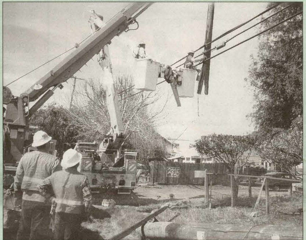
Lineman Steve Hernandez, in the right bucket, removes communications fixtures. Lineman Vick Mahafley observes from left bucket.
