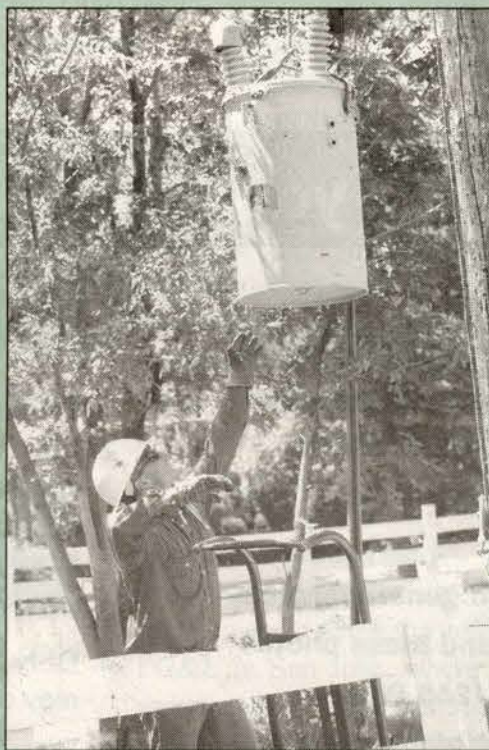
Apprentice Lineman Marc Christensen reaches for the old transformer as it is lowered to the ground.
