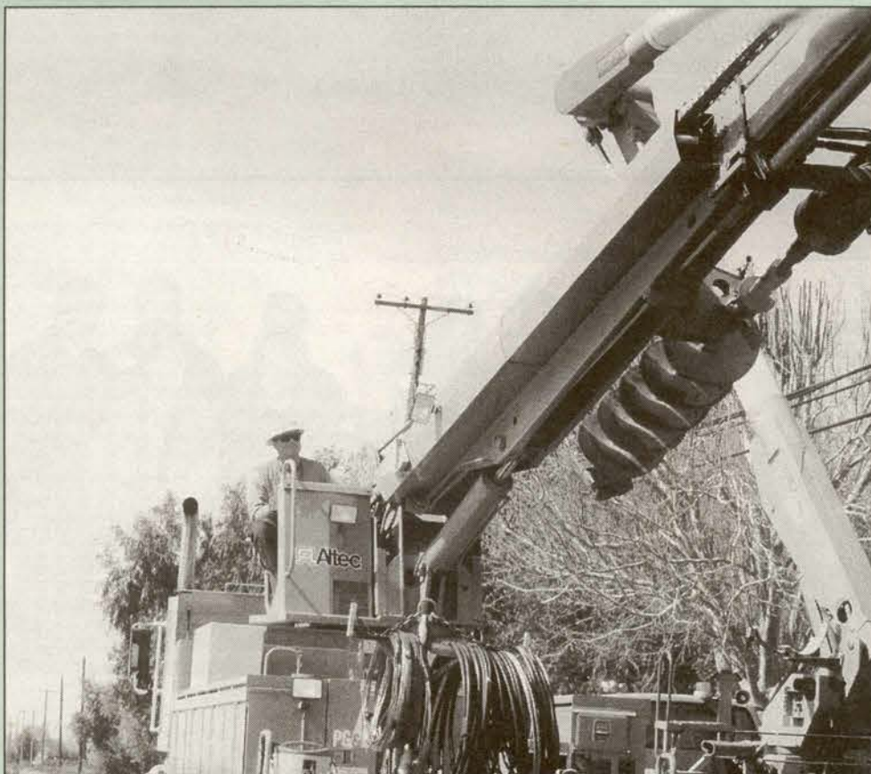
Operating the boom on the line truck is Lineman Jeremy Lehne.
