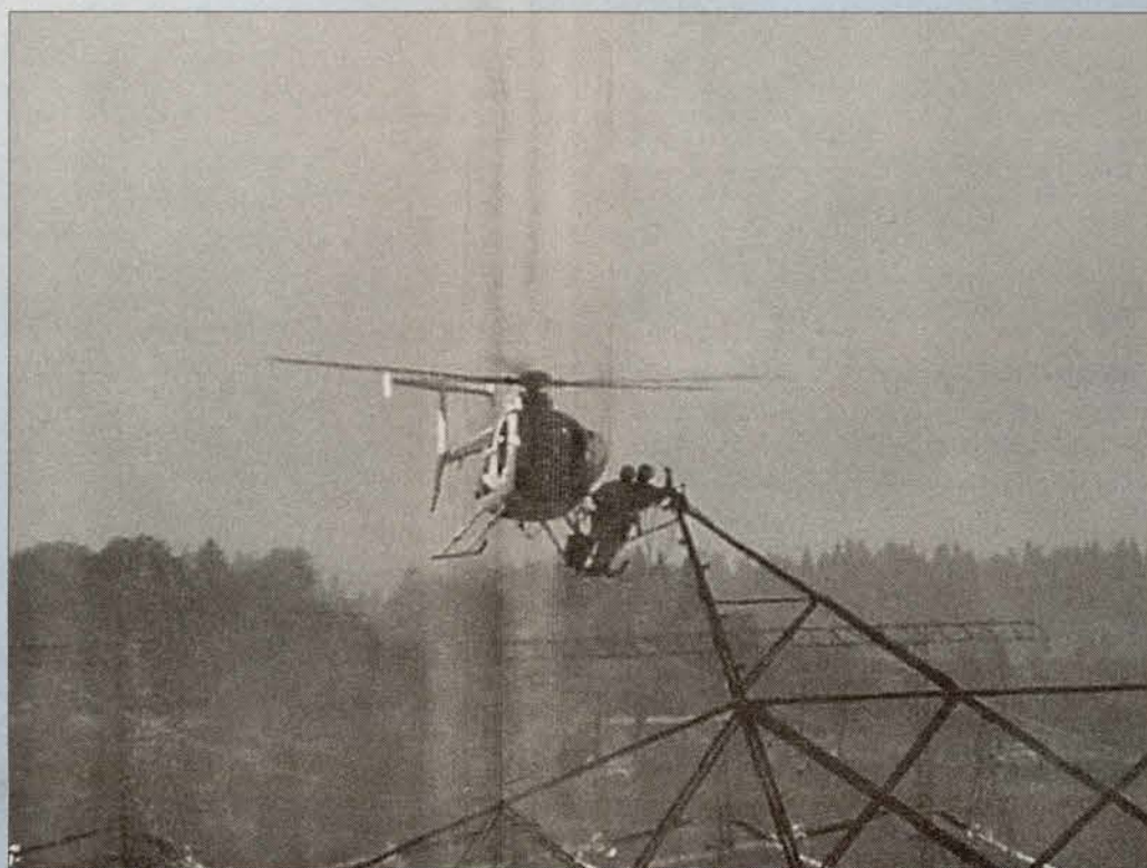
Performing insulator change-out from the skids.
