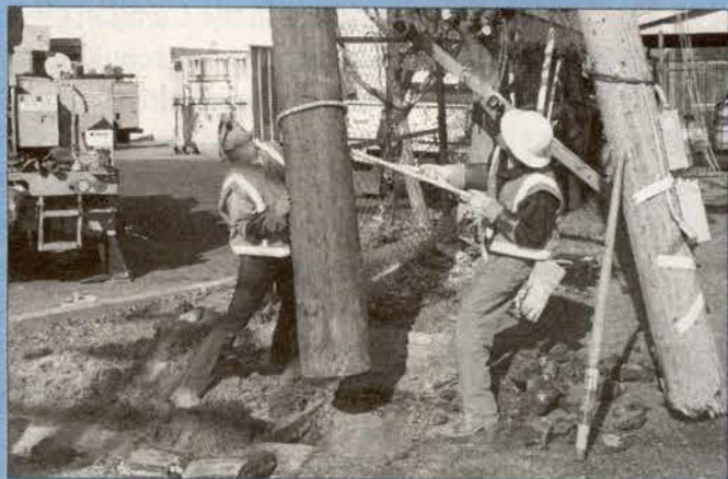
Rotating the pole into position.
