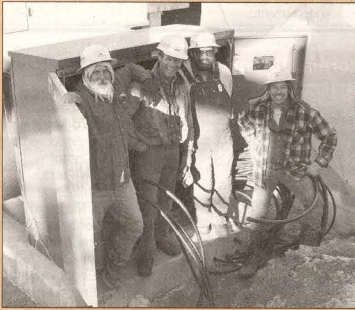
Smily Stahl, Lon Dohnansky, Jack Martin, and Curtis Zahourek next to one of the four 1500 kva transformers they helped build for the project.
