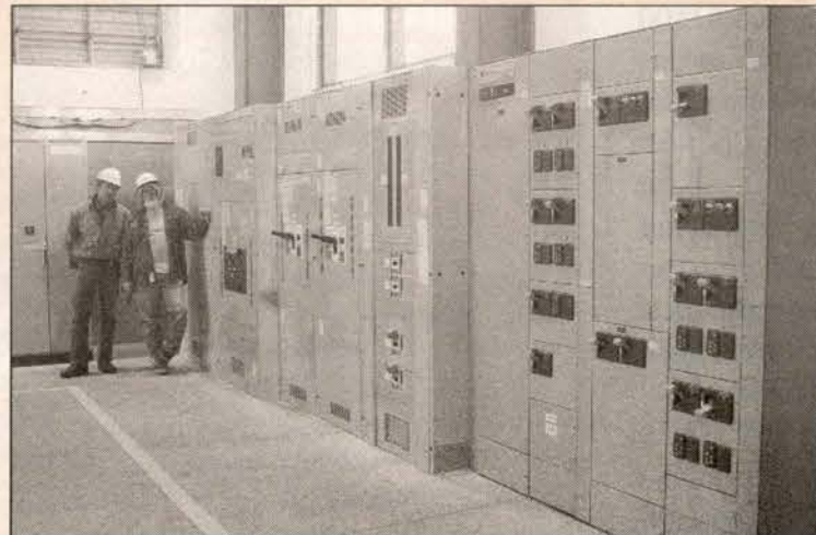
Lon Dohnansky and Smily Stahl in the mountain-top control room built by contractors.
