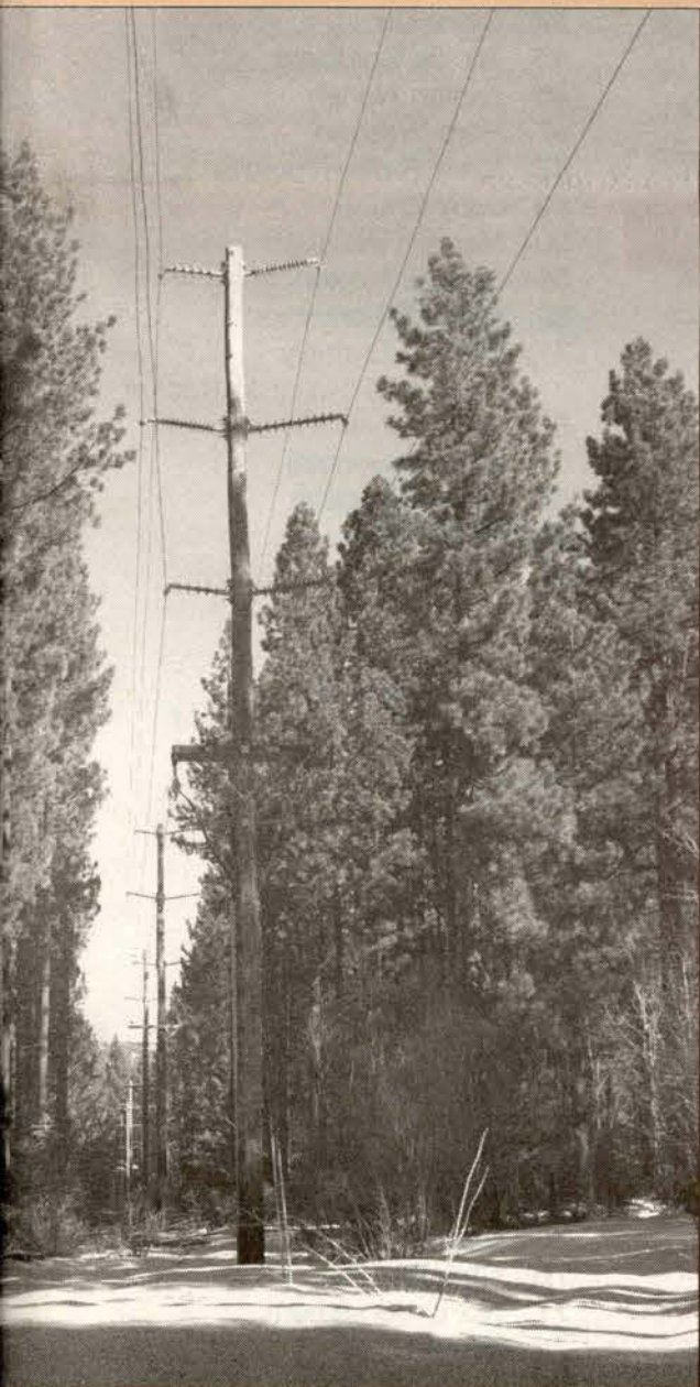
needed to take existing transmission lines like these allow the tram line to pass through.
