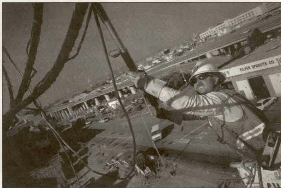
This photograph, part of a series of photos by Local 1245 Lineman Lewis Giles, shows Lineman Dan Goyne at work for PG&E within sight of the Oakland-San Francisco Bay Bridge.
