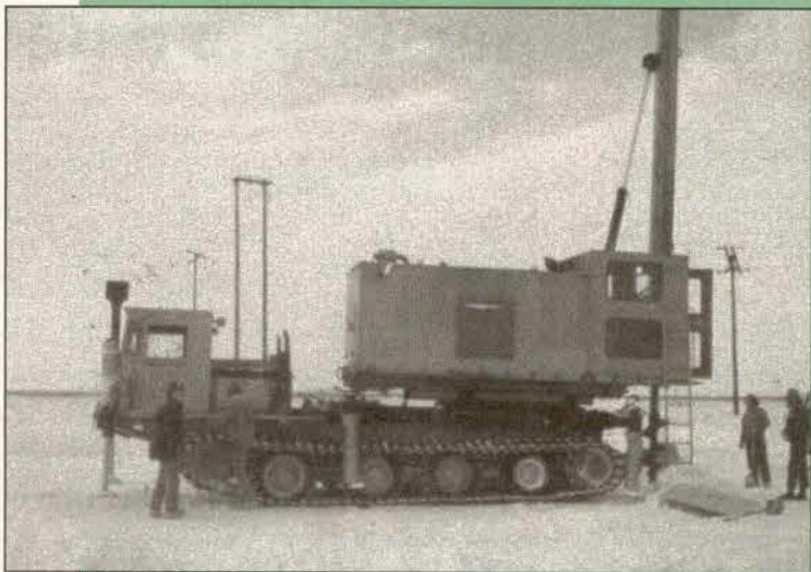
Hole-digging in Arctic permafrost.
