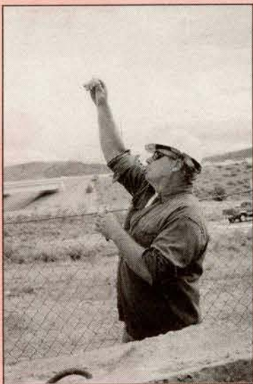
Plumbing the pole.
