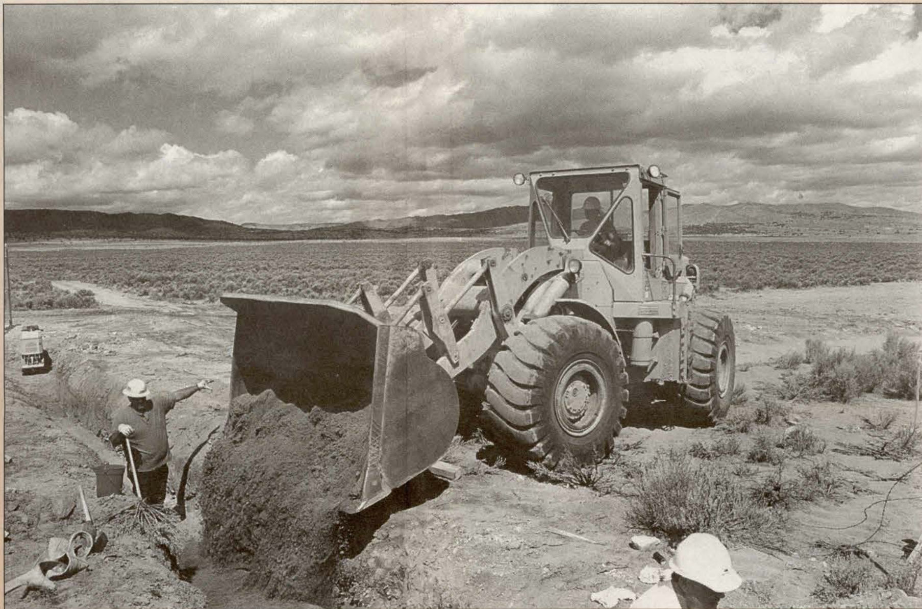
Foreman Tim Lake (signaling) and Tony Lewis.
