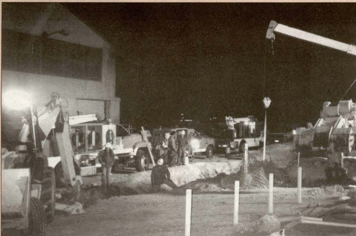
General Construction Welding Crews preparing to align the 36 inch pipe for the final tie-in to the new Turbine Compressors
