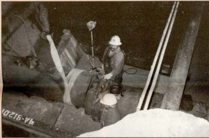
Final fitting of the pipe to measure it for trimming.
