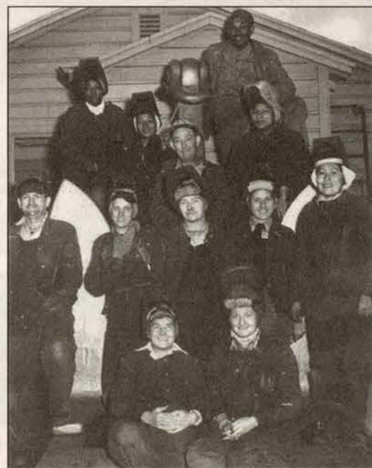
"Peg" Ella Clem and her Yard #2 welding crew. Photo courtesy of Donna Stewart.
