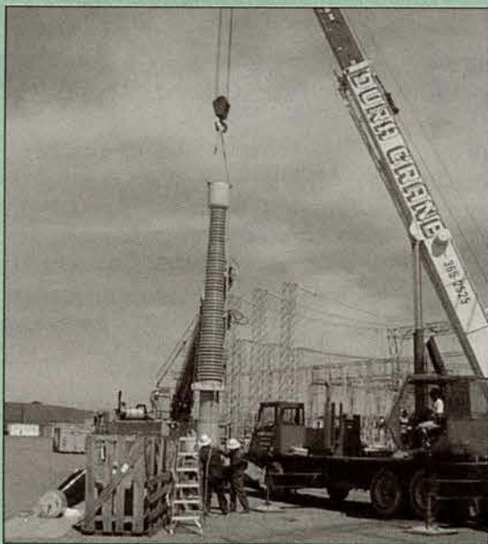
Ron Fargen and Joe Velasquez uncrating new insulation for installation.
