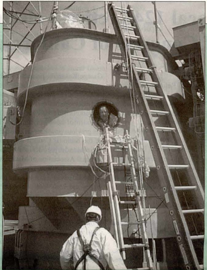
Mike Hamm and Jay Hapitan enter the bad unit to replace blown insulator from inside transformer.
