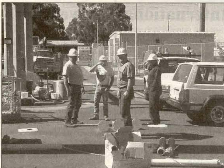
From left: Bob Jesse, PG&E Electric Subforeman A, Bobby Lane, PG&E Working Foreman A, Bill Breeding, SMUD Engineer, Julian Martinez, PG&E Electrician
