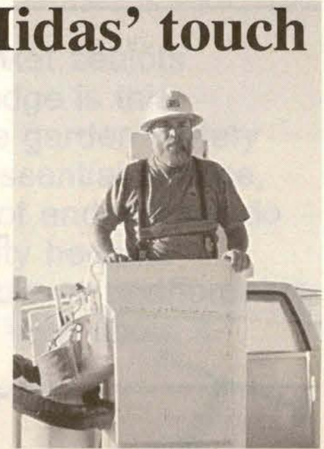
Union steward Santiago Salazar, Substation Construction Control & Testing (SCCAT), working on substation relocation/construction.
