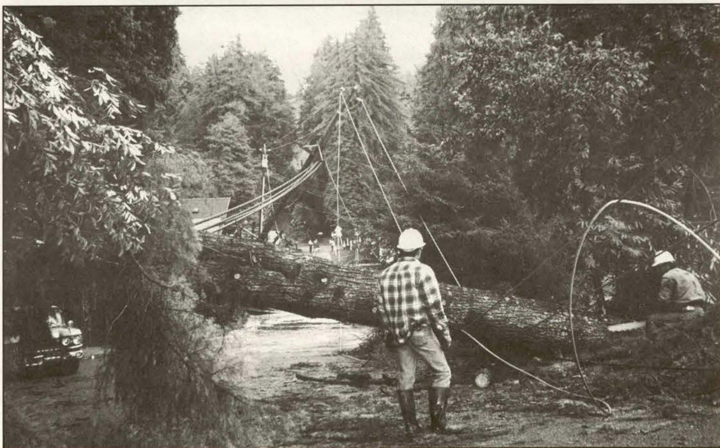
Lineman Don Meyer (above, left) grounds wire before starting work on a fallen line in Sonoma County during the January storm. At left, a Local 1245 crew for Davey Tree removes fallen trees, also in Sonoma County. (Photos: Eric Wolfe)
