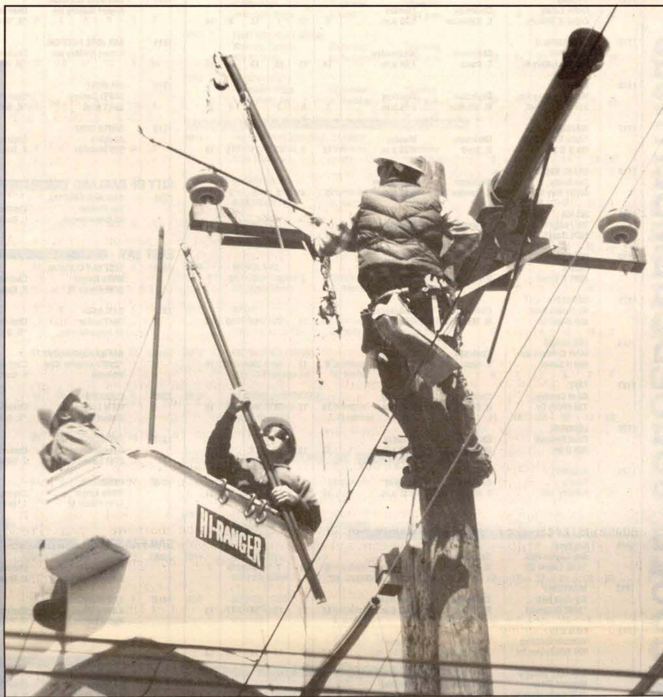
Untying an old 12 KV and lowering it onto a new arm during a job at Clinton and Union Streets in Alameda are, from left, linemen Frank Acala and Bill Tice, and apprentice Jim McRory. (Photos: Eric Wolfe)
