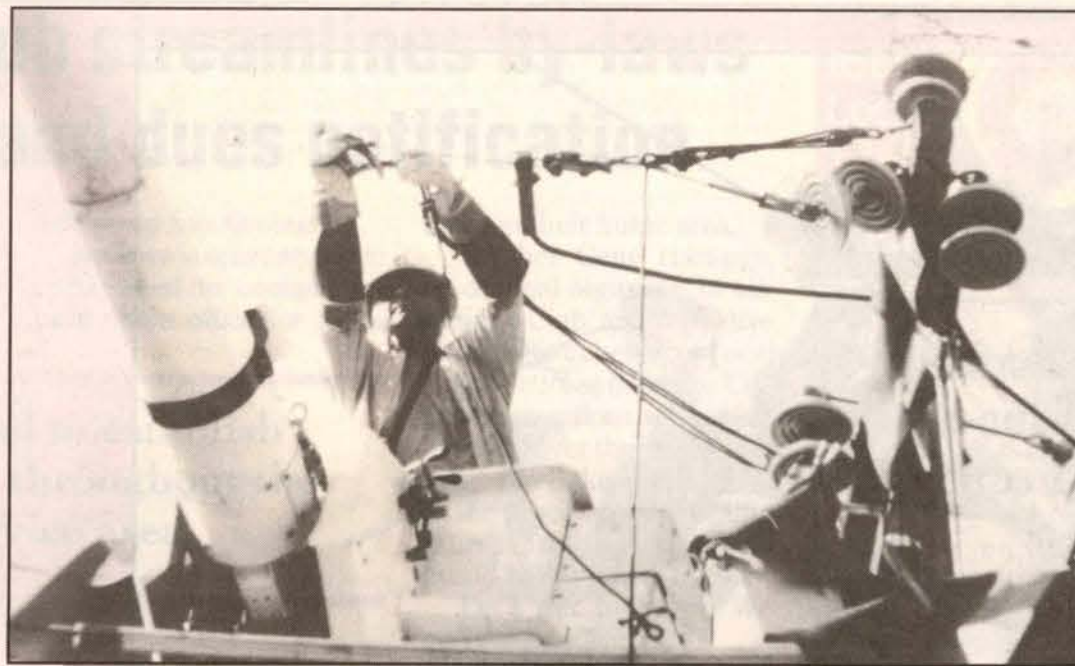
A Local 1245 member wears EMF monitoring gear while rubber-gloving during a pilot study.
