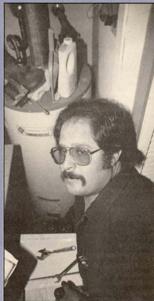
Top: Harold Sheeran (left) and Bryan Wasson repair a gas leak at a South Lake Tahoe apartment complex. Above: Gas serviceman Dave Rust uses leak detector to locate gas leak on the control valve of a hot water heater. Right: Gas serviceman Mike Rosenberg locates leak on hot water heater at a South Lake Tahoe residence.
