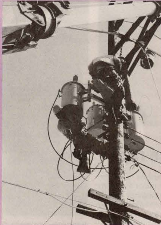
Putting the transformers in place.
