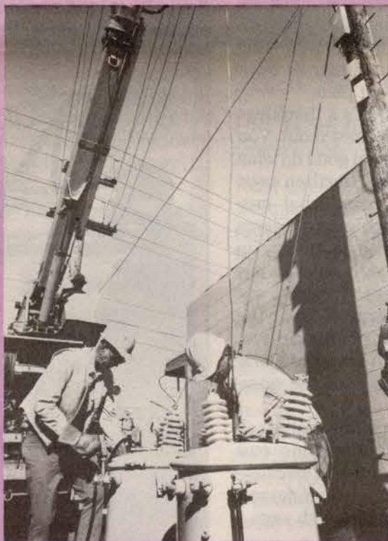
Preparing the transformers for lifting.
