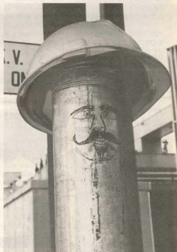
Unidentified member of a SMUD maintenance crew—or is that management?—at Substation A in downtown Sacramento.
