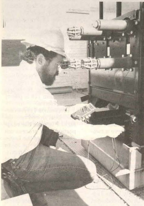
Art Torres, shop steward, running tests during maintenance on 12kv air circuit breaker.
