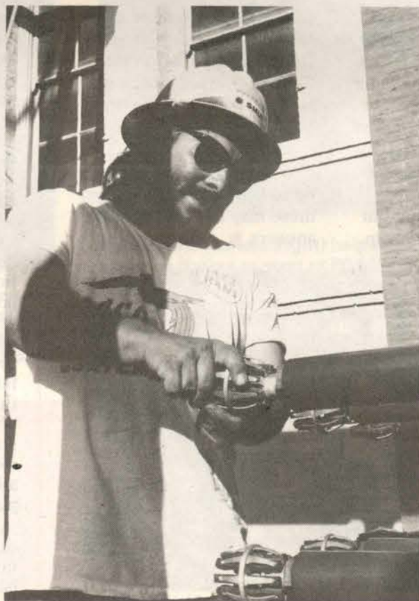
Frank Hernandez, 15-year union member, cleans the "tulips," the connections that go into the bus.
