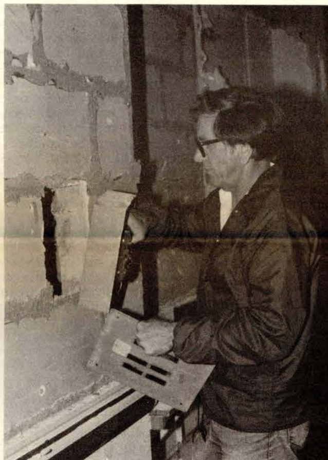
Jim Krugh, Electrician Leader, removes old circuit breaker.
