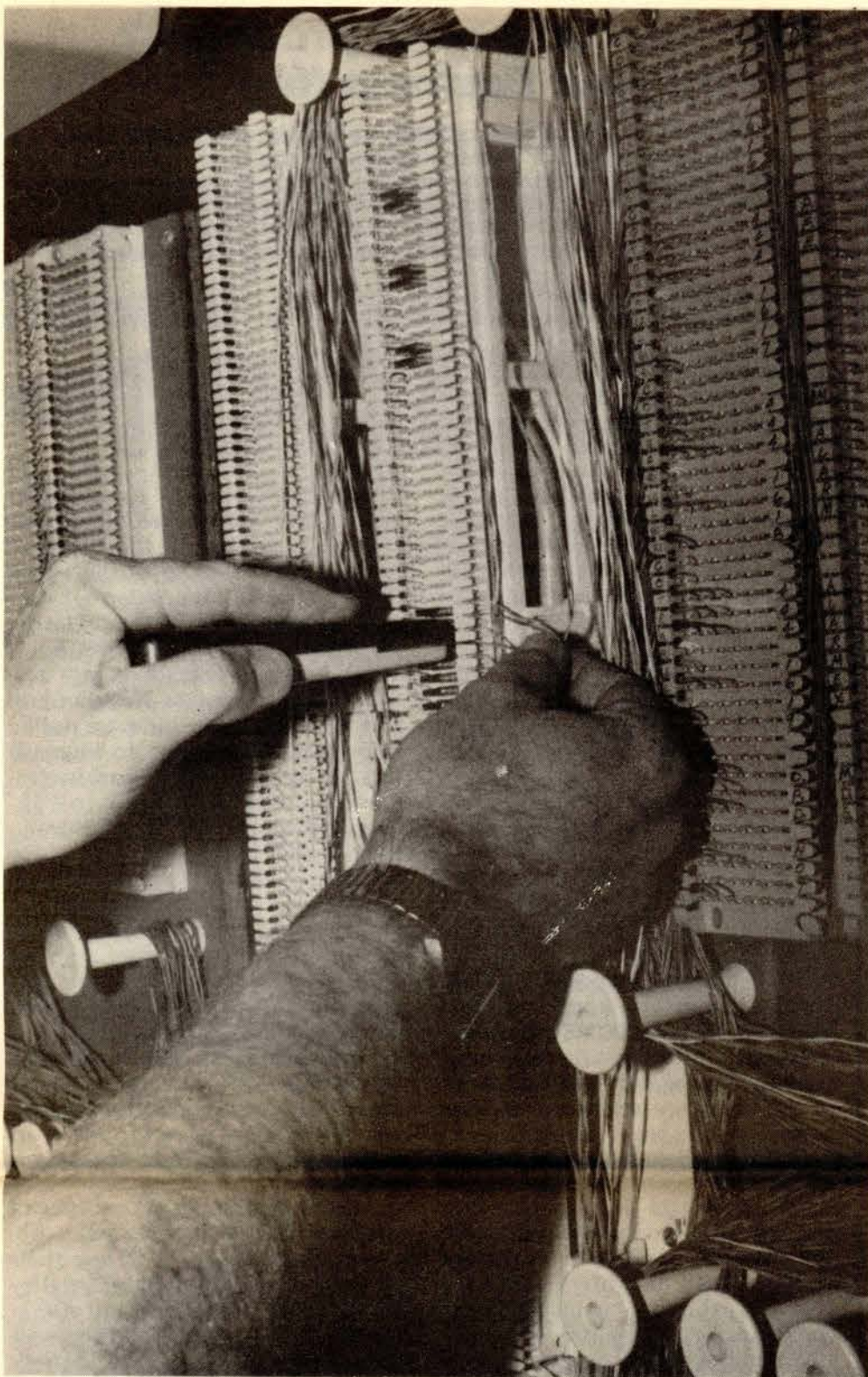
Circuit being connected.
