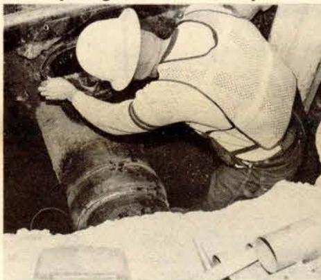
Soap testing the weld.
