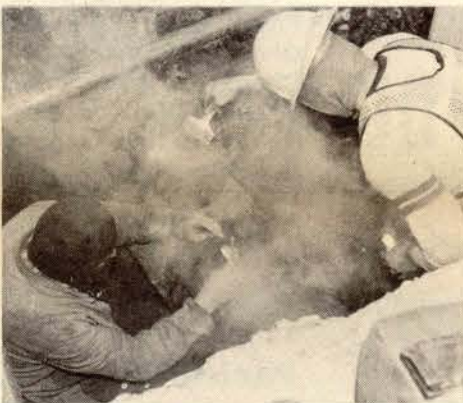
Soap testing the weld.
