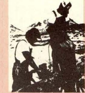
Draper, Arla, Haynes prepare to connect hardware on pole which is framed on the ground.
