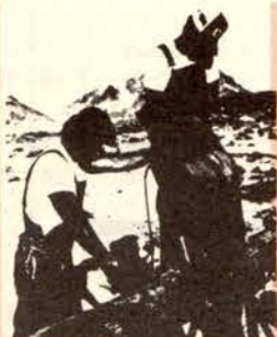
Draper, Ariz. Haynes prepares to connect hardware on pole which is framed on the ground.
