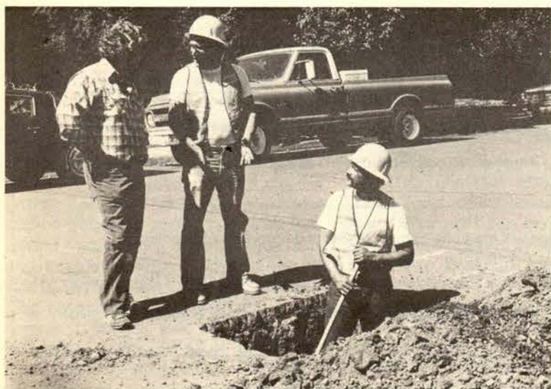
Gibbs in field with Unit Chairman Bettencourt, a Fitter, center, and co-worker, Mike Martin, Temporary Fieldman, who are working on locating and repairing a gas leak.
