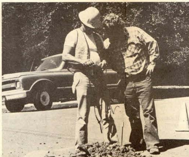
Bettencourt shows Gibbs how 'sniffer' helps pinpoint gas concentrations.
