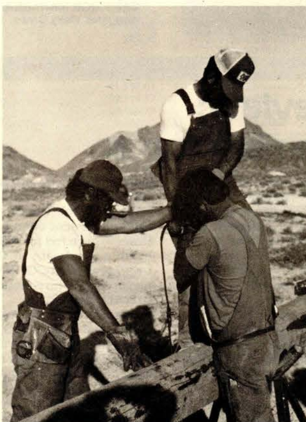
Draper, Arla, Haynes prepare to connect hardware on pole which is framed on the ground.
