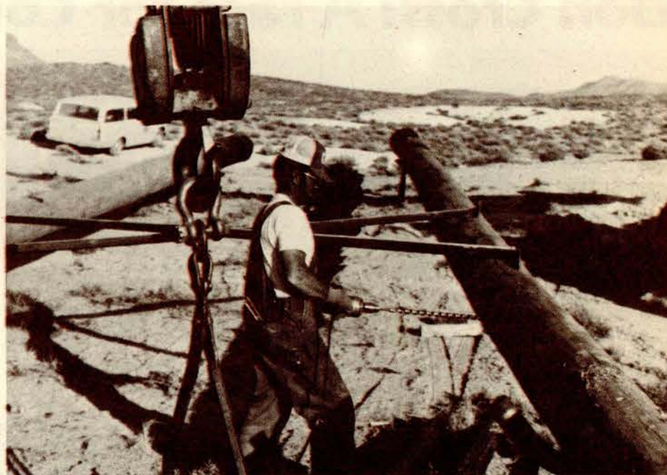
Working Foreman, John Arla, Reno; drills hole in preparation of framing pole.
