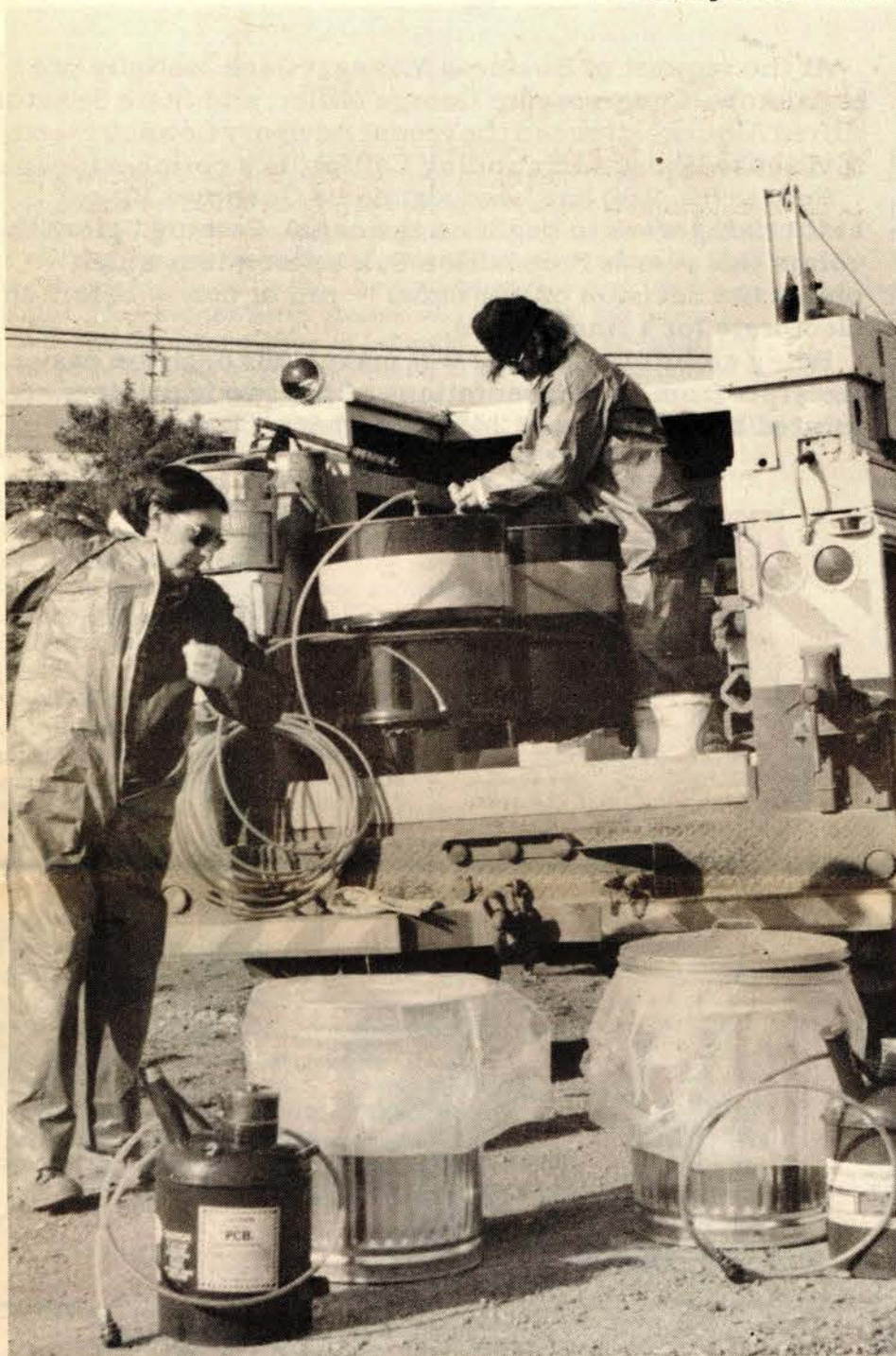
Al Amodeo, left, and Helper Dale Lachappelle, right, put on protective clothing and ready safety equipment needed to pump oil out of gas line.
