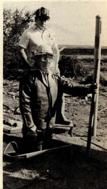
Al Amodeo, foreground, removing oil with possible PCB contamination out of the gas service line.
