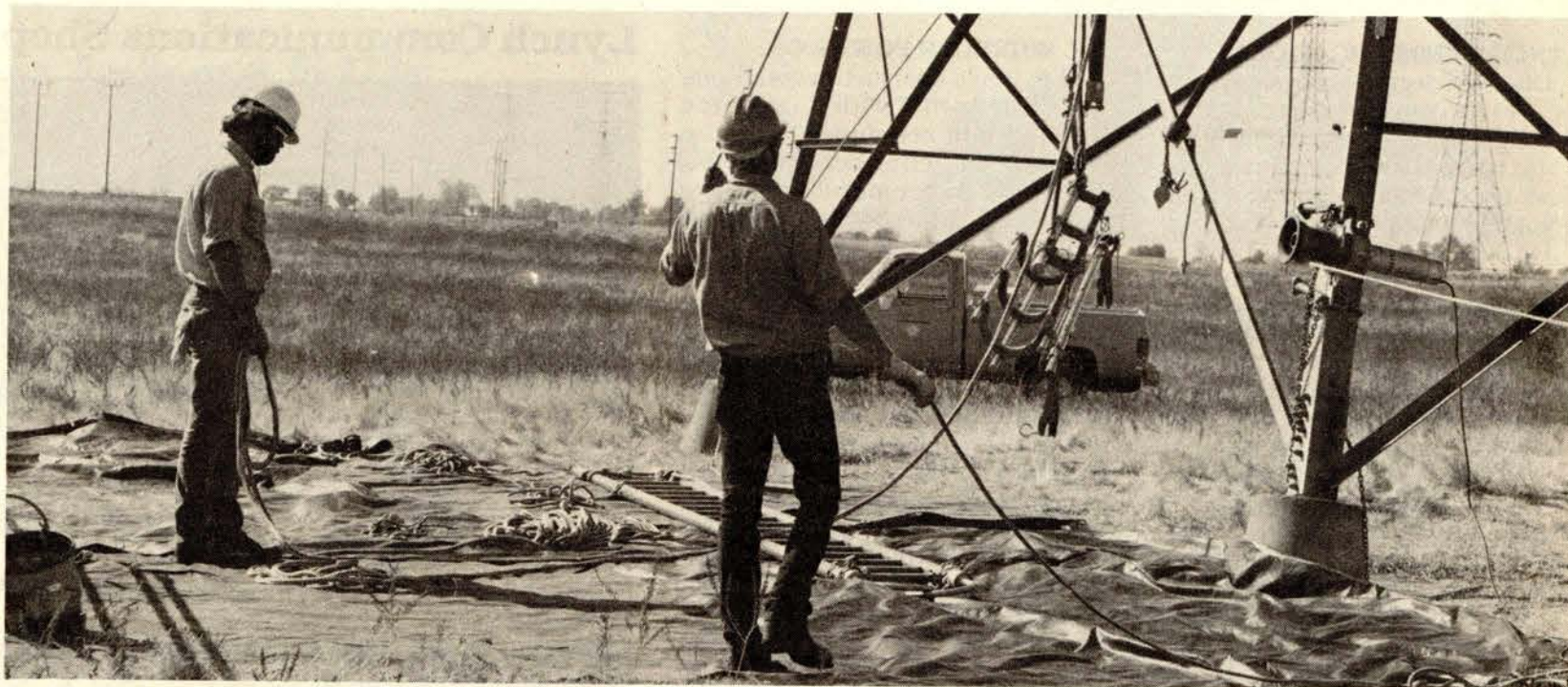
Readying mobile insulated boom to be hoisted up the tower are Linemen Mike Eckhardt, left, and Dennis Jorgensen.
