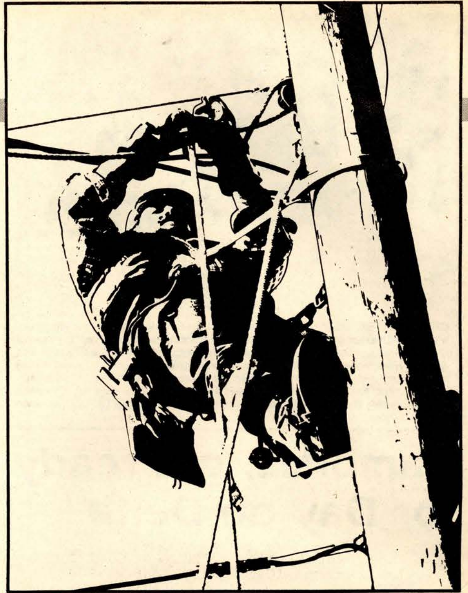
WORKING HARD... Shop Steward Dave Pittman, Modesto Irrigation District Lineman, replaces wires.
