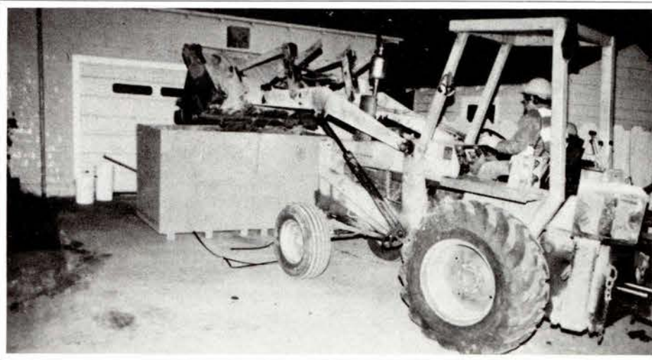
Backhoe Operator removed contaminated soil and materials to deposit them into company supplied contamination boxes.
