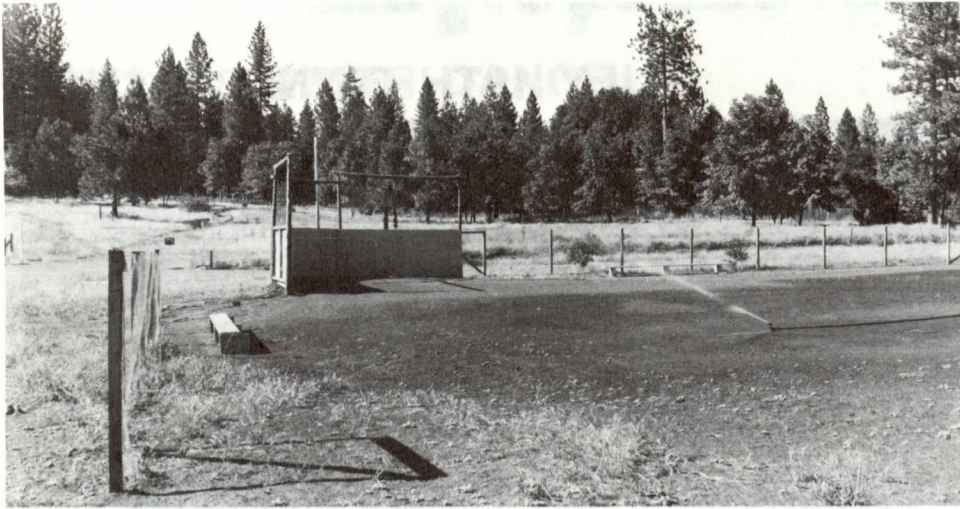
This photo shows the practice field built by Local 1245 members and others in the community.
