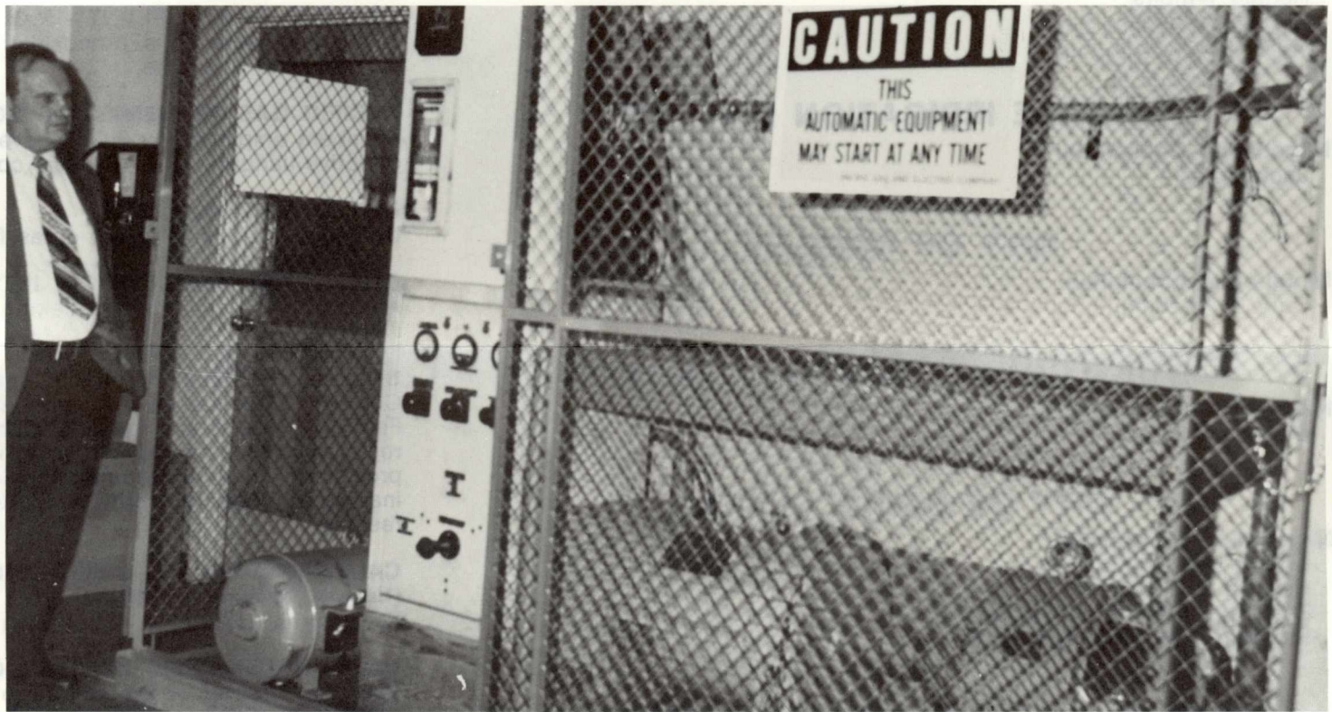
Jack Allen, instructor, is at the Generator Control Board and synchronizing panel to demonstrate the start up of the simulated Hydro Plant.
