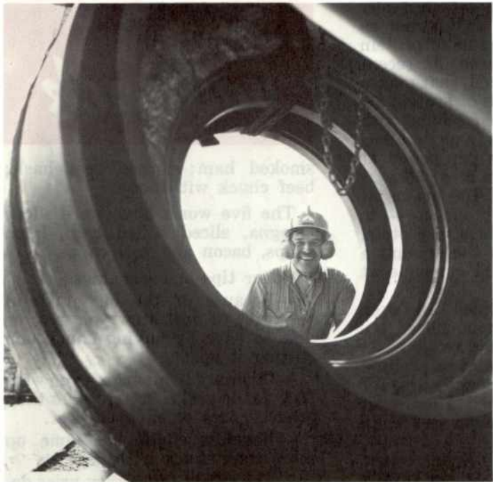
This photo shows Truman Bates removing volute of Unit B compressor, Station #13, just east of Crater Lake, Oregon.
