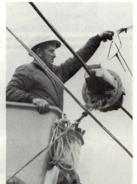
Dan Cribur, lineman, is shown working in "bucket truck."
