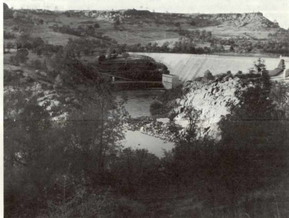
This photo shows Tulloch Dam, power house and part of the afterbay.
