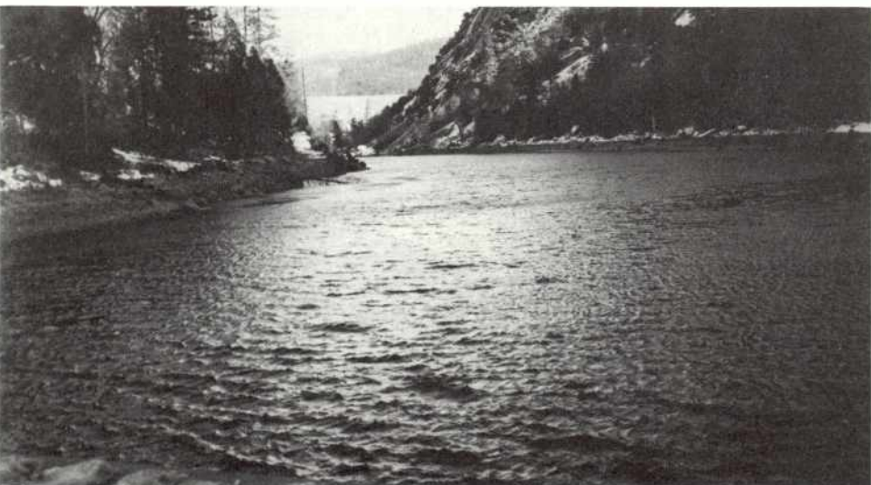
Beardsley's timber-crib and rock afterbay provided the footing for this photo.
