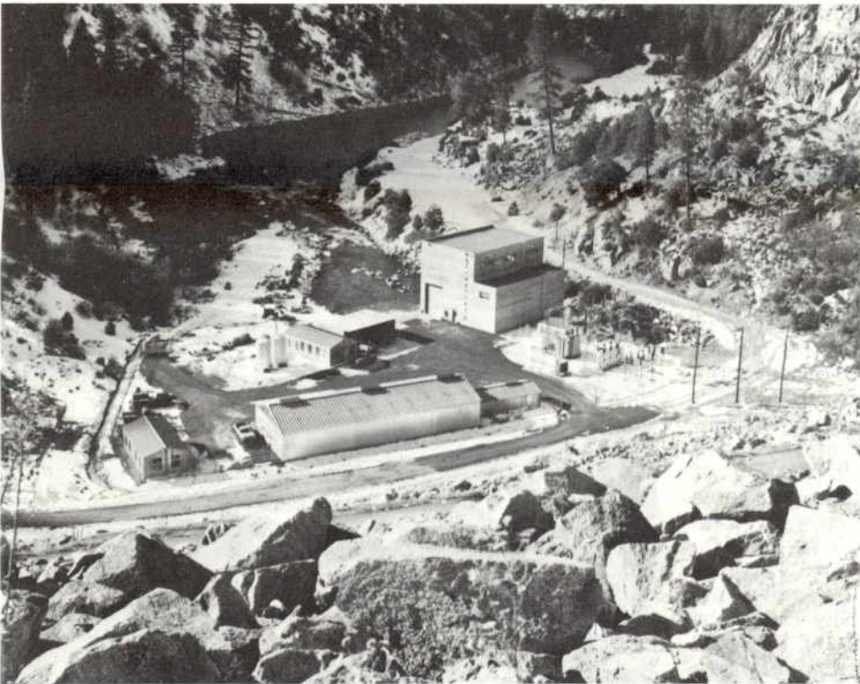
This view of the maintenance shop, power plant and Beardsley afterbay was taken from the top of the dam.
