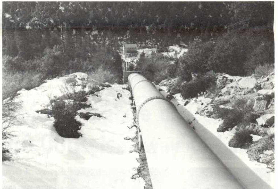
This photo shows the 0.5 miles of 81' diameter penstock which delivers the water to Donnells power plant.
