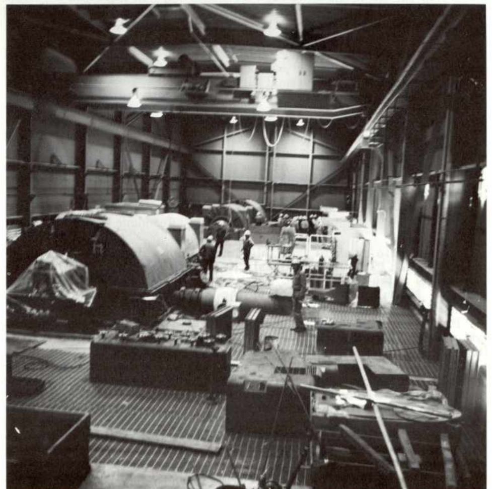
The photos above and below show the complete structure, inside and out, of units 5 and 6 of Pacific Gas and Electric Company's The Geysers Geothermal Power Plant in Northern California. Unit 6 was being tested the day we were there, and is shown in the photo above this one. When both units go into commercial operation late in 1971, they will bring total plant production at The Geysers to a capacity of 192,000 kilowatts. Units 5 and 6 house the world's largest geothermal steam turbine-generator units, which are shown in the photo below.
