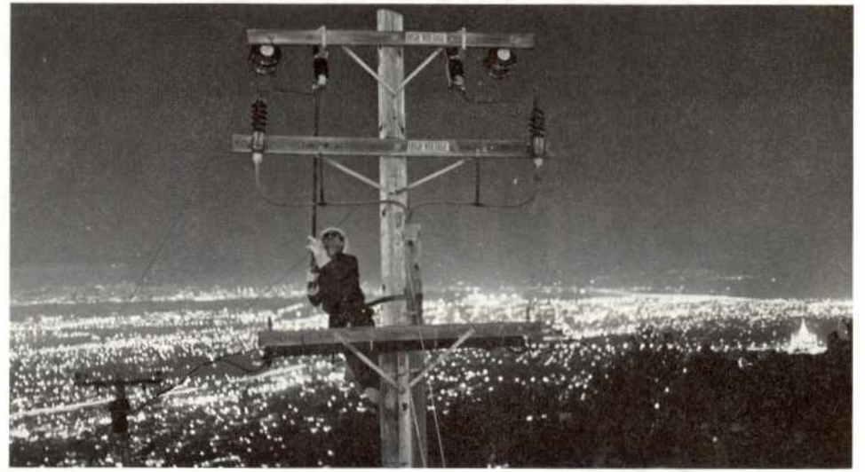
HOT STICK ON A HIGH LINE —By using tools attached to slender poles, PG&E troublemen like Jim Mosser, who's shown working high atop an Oakland hill, often repair energized or "hot" electric lines. The "hot stick" work avoids power interruptions and has helped PG&E achieve a nearly perfect reliability index.
