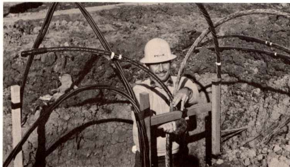
Henry Corrales, Working Foreman in the Gas Dept., G.C. and Shop Steward, is shown tying up underground cable in a joint-trench in a San Jose subdivision.
