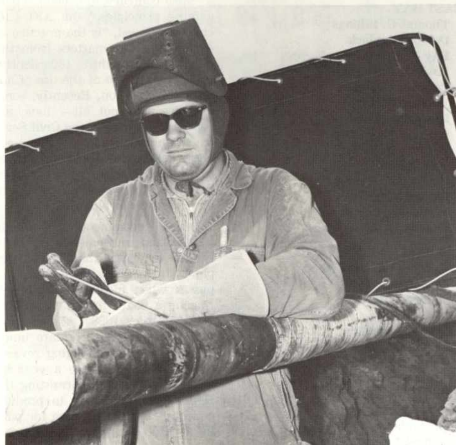
Bernie Tanksley, working as a Mechanic, is just about to pull his welder's mask down before striking an arc on a 4 inch high
