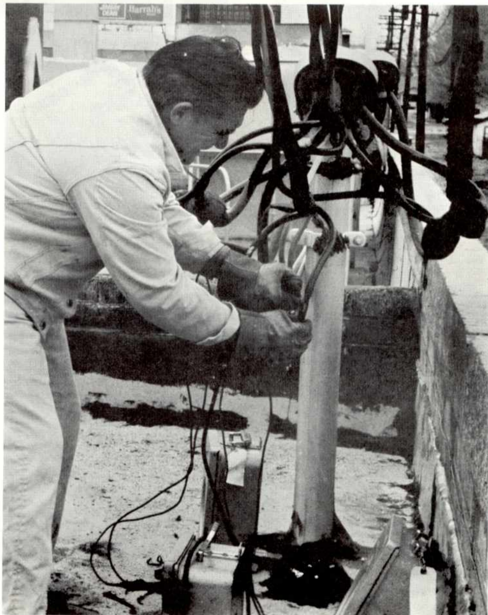
Troubleman Nick Danos tests voltage on a rooftop.
