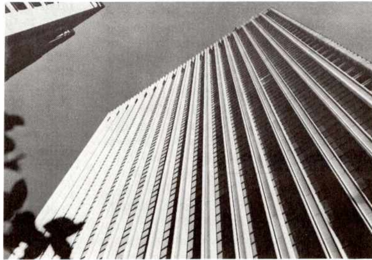
"Where or where has my Cartman gone?" wails Cable Splicer Patterson. "To the top of the new Wells Fargo building to complete installation of transformer banks" (underground jurisdiction here extends 43 stories up, please note), says the Cartman, hastily grabbing another view of The City.
