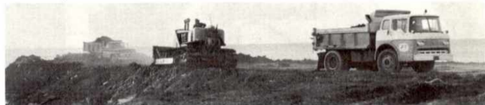
The trucks bring their dirt to the foot of Ashby Avenue, and the bulldozer pushes it into the waters of San Francisco Bay. This particular dump job was started after September 17th, the effective date of the Bay conservation and development legislation authored by State Senator Eugene McAteer. This leg of fill is intended to circle out and join a mile or so offshore with another dump job which has been going on for several months from the foot of Powell Street.
