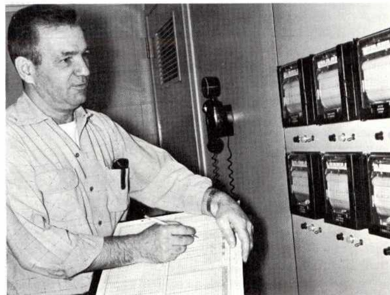
In the San Jose Gas Load Center, Pressure Operator Sam Clark records the chart readings.
