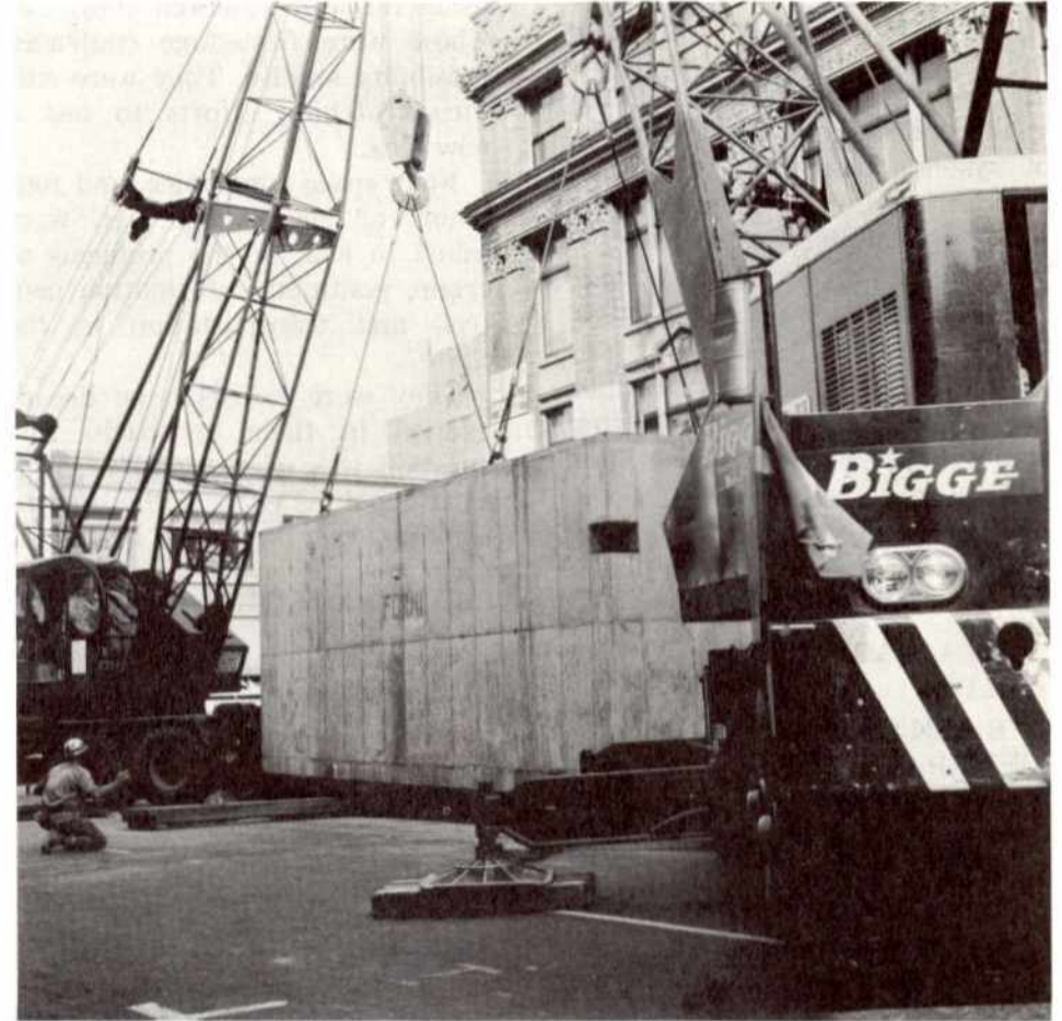
7. Lower away! Note the Bigge employee crouching at left, directing his crane operators with hand signals and whistles. Manufactured by the Forni Corporation of Oakland, the transformer vault is large enough to house two 12,000 volt transformer banks, complete with switchgear and downtown distribution-network protector units.
