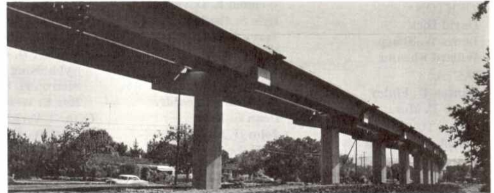
A completed portion of elevated track in Concord.
