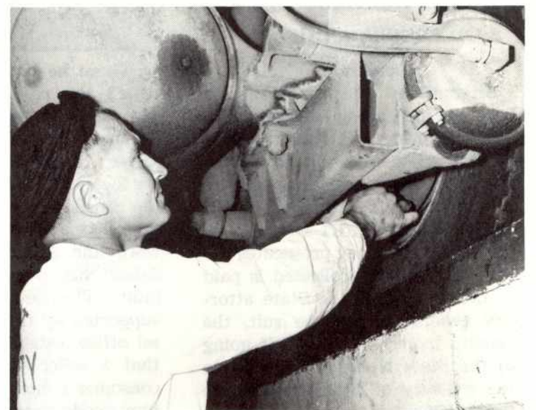
2. Bob Calzascia, Advisory Councilman for the Transit Authority of the City of Sacramento, checks the rear axle assembly on a GM TDH-4519 Transitliner.
