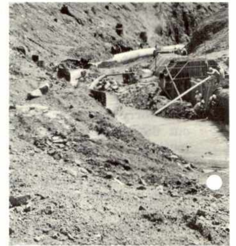
The Iron Canyon diversion construction.
