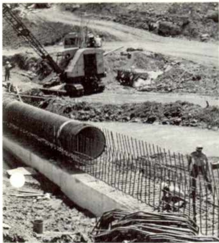
n tunnel shown under con-
