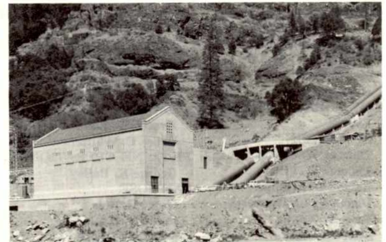
This is Pit 4 Powerhouse.
